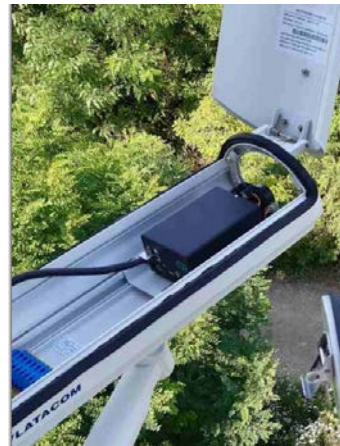
Figure 6. An IP camera in an outdoor enclosure during the installation
