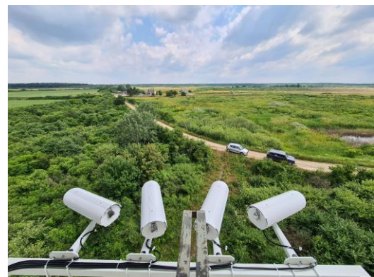
Figure 15. View from watchtower with installed cameras
