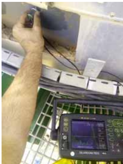
Figure 3. Display of ultrasonic thickness gauge during wall thickness
