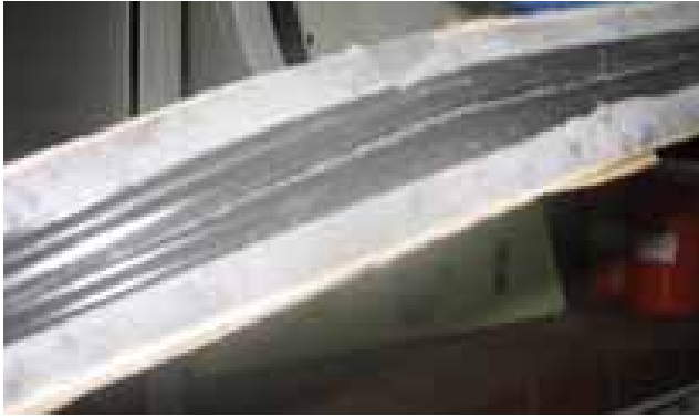
Figure 5. Cracks in the grain channel
