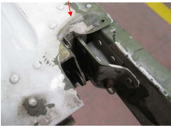
Figure 12. Deformed skin of the horizontal stabilizer
