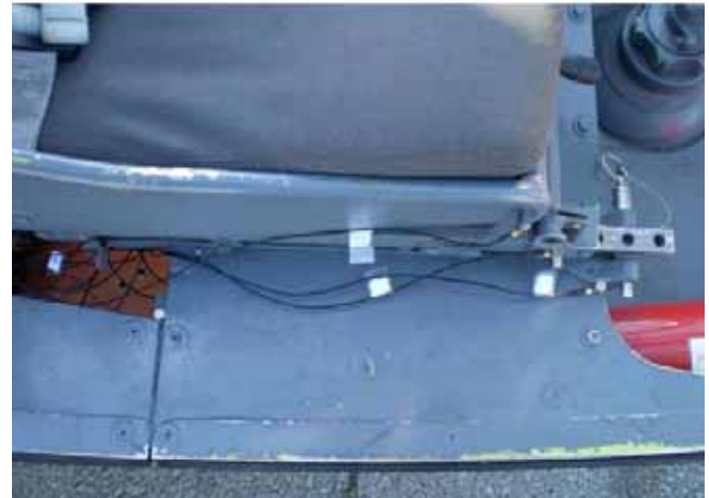
Figure 4. Equipment installed on specific locations in the cabin floor for flight testing
