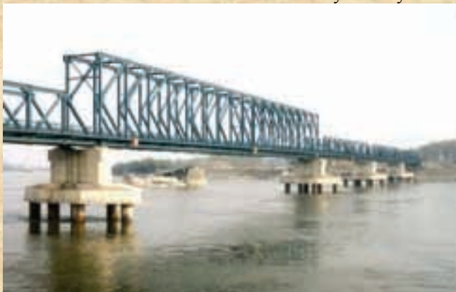
Figure 47. MД-88 Bridge over the Danube near Novi Sad
