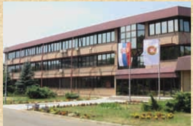
Figure 2. Current VTI management building in Žarkovo
