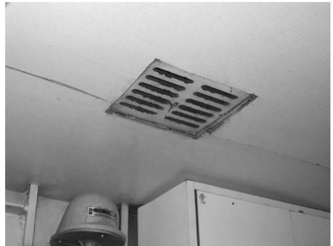
Figure 5. Ventilation opening with air flow regulation in the corporal cabin
